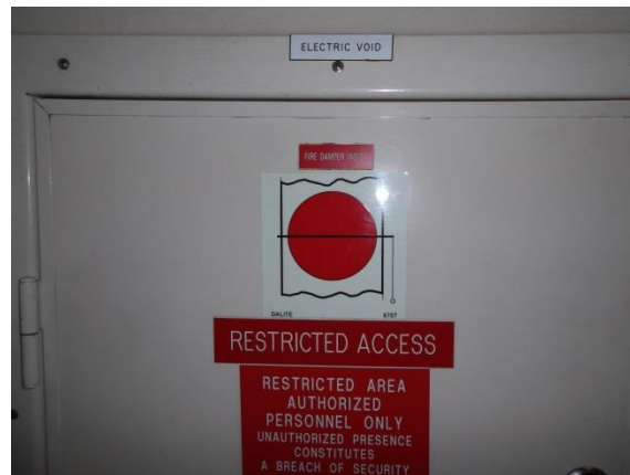
Figure 10: Example of “Restricted Bridge Access” Placard
