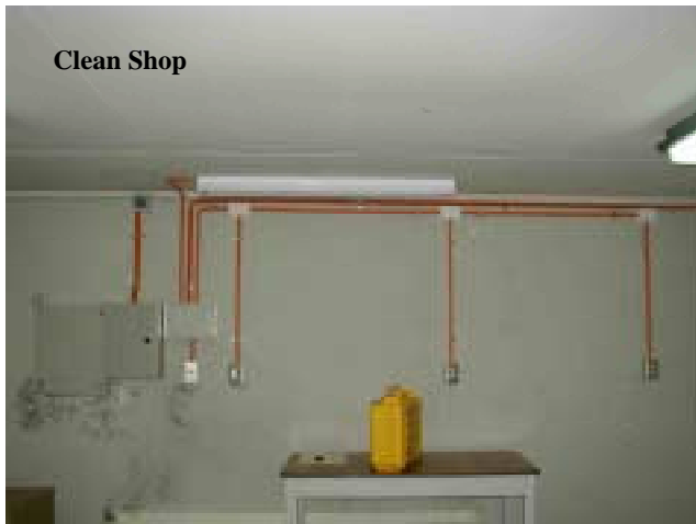
area New electrical power outlets at warehouse
