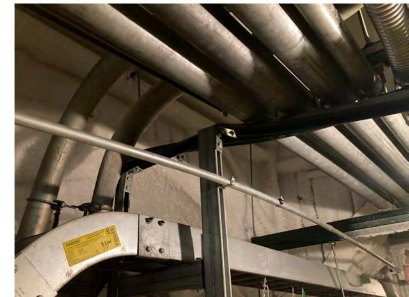
Fixed point connections experiencing deformation due to ice sheet movement.
